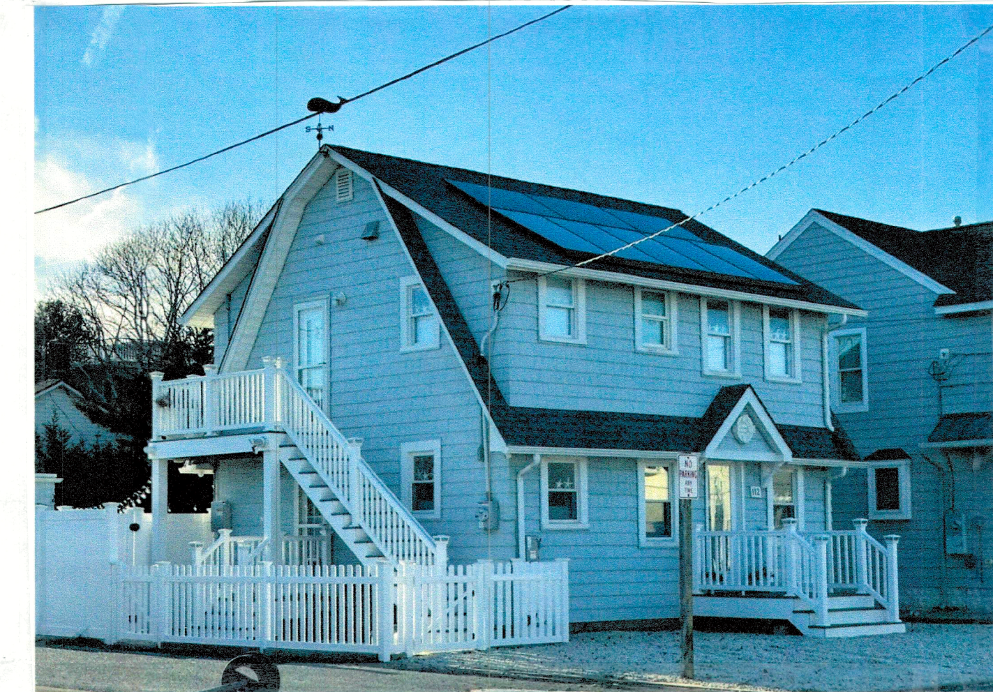
PHOTO OF EXISTING DUPLEX SHOWING EAST AND NORTH SIDE ELEVATIONS
